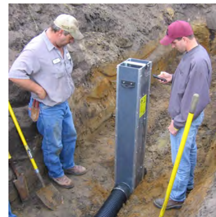
Stop Log Structure
